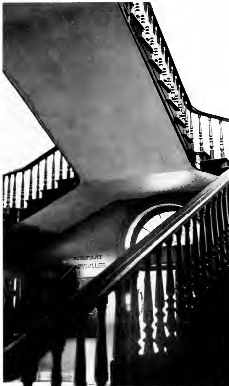
FIGURE 21. Double flight of stairs designed by William Strickland for the Second Bank of the United States in Philadelphia (compare to stairs shown in figure 20 ). Courtesy of Library of Congress, Prints and Photographs Division, HABS, PA, 51-PHILA, 223-34.
