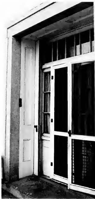
FIGURE 19. Front door, with granite crossetted architecture, Berry Hill Plantation house. Courtesy of the Virginia Department of Historic Resources, negative no. 15859, frame 31-A.
