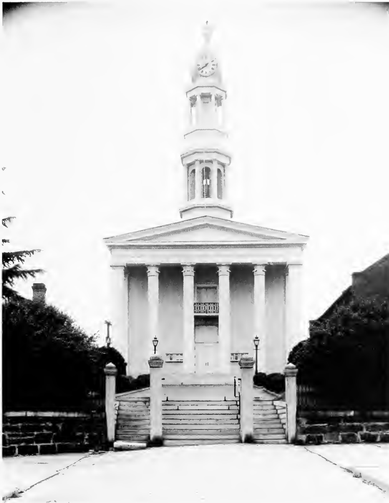
FIGURE 6. Court-house, Petersburg, Virginia, commissioned in 1838. Calvin Pollard, architect. Courtesy of the Library of Congress, Prints and Photographs Division, HABS, VA,2--PET,29-2.
