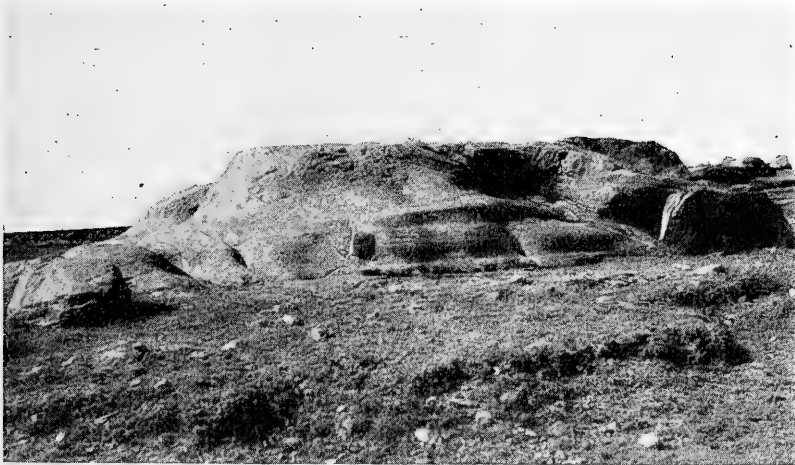
FIG. 15.—View showing recent uncovering of grooved granite
