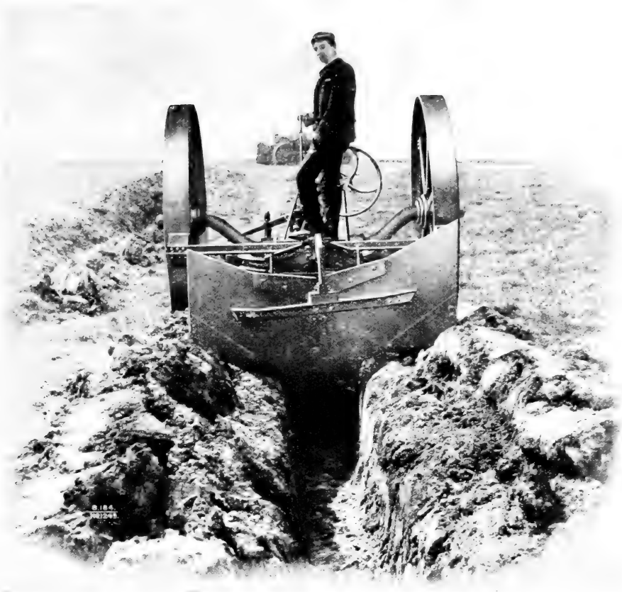
FIG. 12.—Fowler Trenching Machine at Work.
