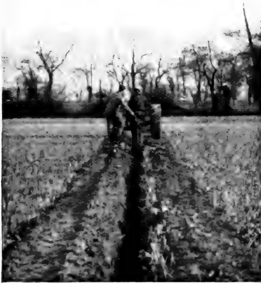
FIG. 6A.—Swedish Excavator and Fordson Tractor, Rear View.
