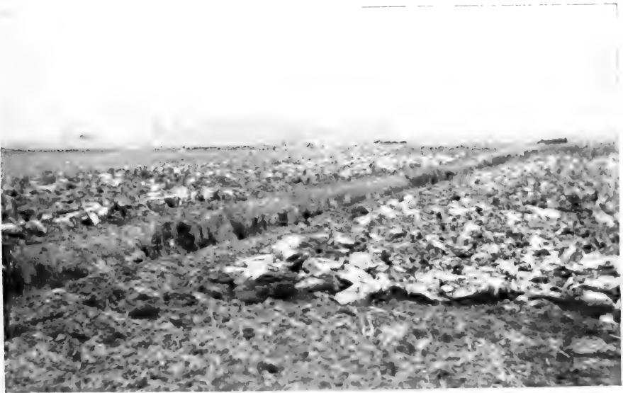
FIG. 2.— The Clay spread, and Trench ready for filling in.
