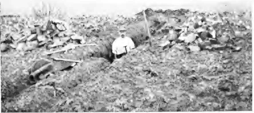
FIG. 1.—Digging the Clay, which is 4 ft. below the surface.
