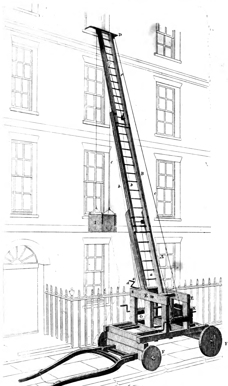
Mr. Davis's Fire Escape
