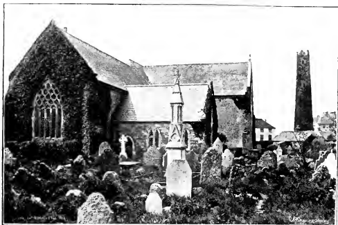
Cloyne Cathedral, N.E. View.
