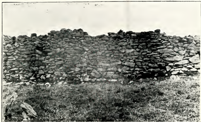
CAHIRCONREE: VIEW OF WALL FROM THE OUTSIDE.
