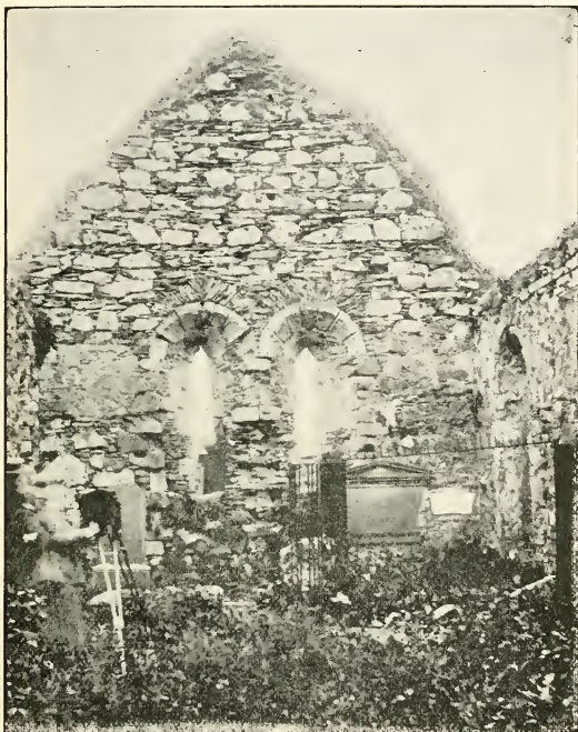
East end Interior of Kildalton Church.
