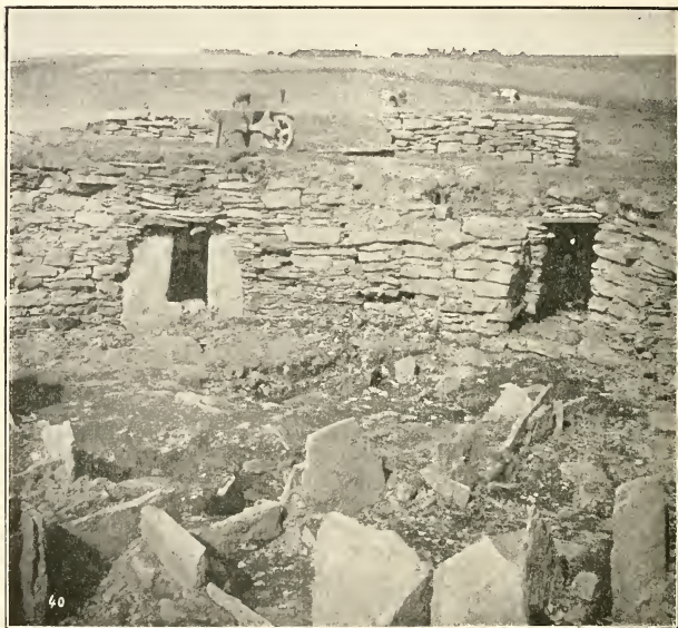
Keiss Road Broch. Interior, showing entrances to Chambers in thickness of wall.
