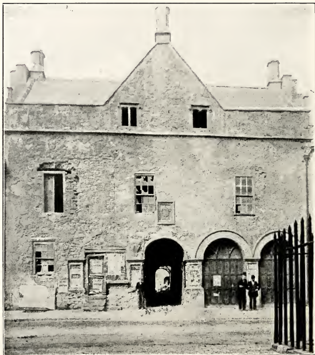
FRONT VIEW OF ROTHE'S HOUSE, PARLIAMENT-ST., KILKENNY, IN 1898, After the roof and chimneys had been restored, but before the front had been renovated.
