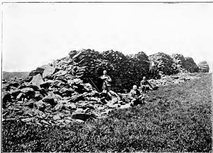
CAHIRCONREE: OUTSIDE OF WALL, LOOKING NORTH-WEST.
