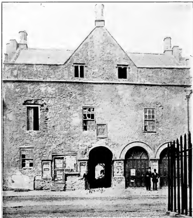
FRONT VIEW OF ROTHE'S HOUSE, PARLIAMENT-ST., KILKENNY, IN 1898, After the roof and chimneys had been restored, but before the front had been renovated.
