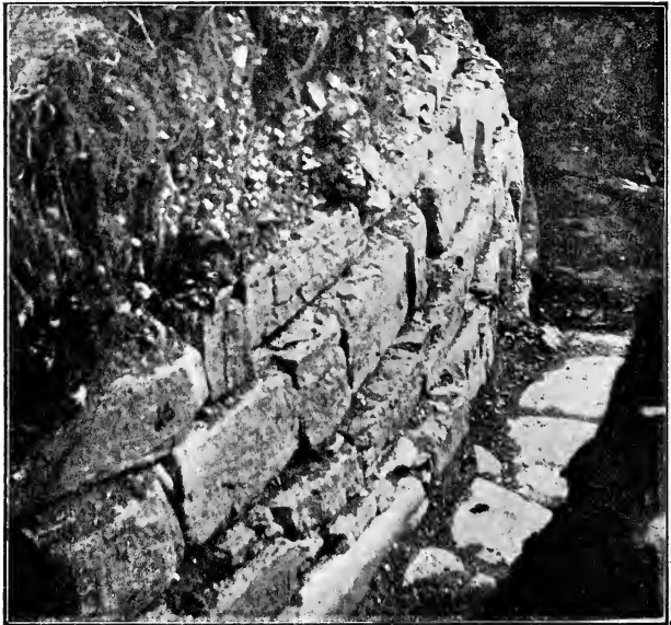
Keiss Road Broch. Foundation courses of exterior wall of older structure.
