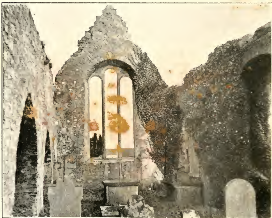
EAST WINDOW OF SOUTH CHAPEL (INTERIOR) DULEEK
