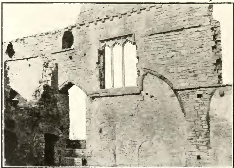
FIG. 2.—BECTIVE ABBEY: SOUTH WALL OF NAVE
