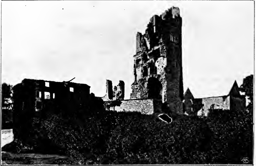
DESMOND'S CASTLE, ASKEATON, FROM NORTH
