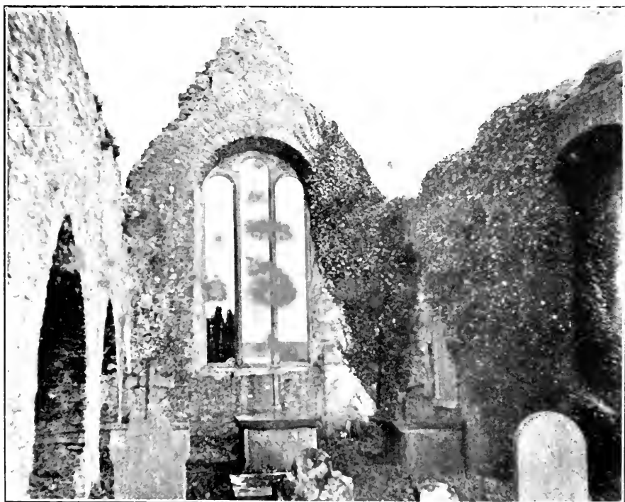
EAST WINDOW OF SOUTH CHAPEL (INTERIOR) DULEEK
