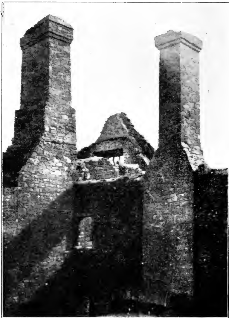
CHIMNEY STACK, BECTIVE ABBEY
