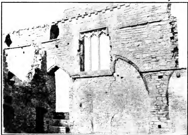
FIG. 2.—BECTIVE ABBEY: SOUTH WALL OF NAVE
