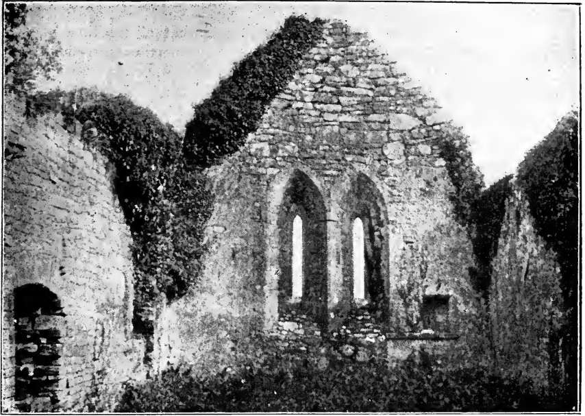
Teampul Mor—Interior, looking East
