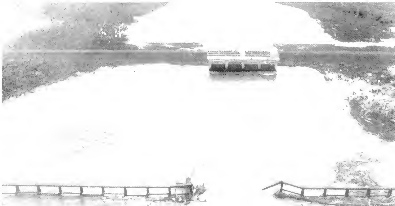
Figure 6. A controlled freshwater diversion structure located on the lower Mississippi River.
