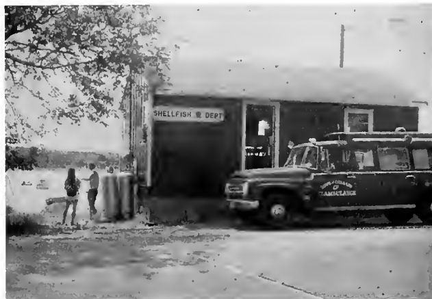
Figure 6. A 16' × 24' (5.1 × 8 m) building was moved to the shores of Town Cove where a seawater system was installed. Within 2 years after moving the building, the town constructed a bulkhead that substantially enhanced the area for recreational boating. This led to incompatibility with the shellfish lab.
