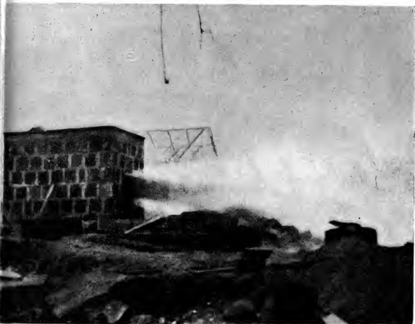
FIG. 4. The 1915 film vault test to determine proper vent area; no sprinkler protection. This small test vault contained 1900 pounds of film, mostly in containers. Vent area was standard. Blow torch flame shown was 8 feet in diameter, extended 70 feet, and lasted about 90 seconds.
