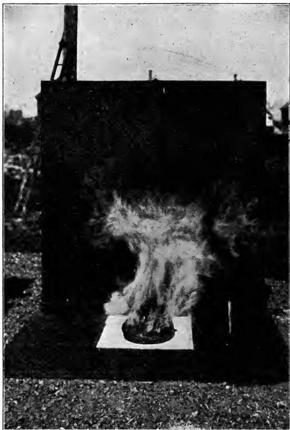
FIG. 1. Film decomposing. Note large volume of gas evolved.
