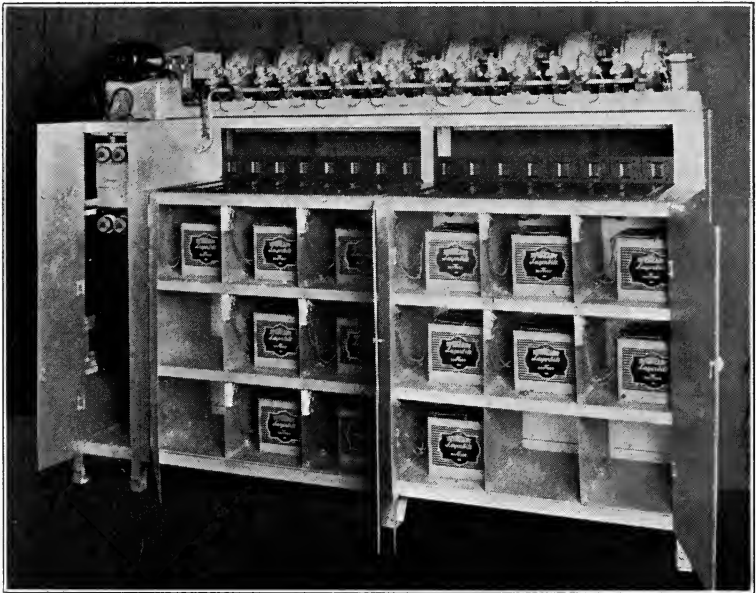
FIG. 1. Call-announcing apparatus with covers removed. At the top can be seen the driving motor and the 8 drums, each bearing 8 strips of film. Associated with each strip of film is an exciting lamp, optical system, and photo-electric cell.
