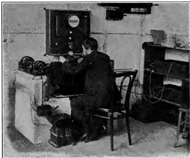
FIG. 4. View of recording apparatus. The driving motors are mounted on a base adjacent to the apparatus proper. Above is the speed indicator for the synchronous motor. The operator observes the recording through the focusing microscope. His left hand rests on the lever that disengages the coupling between the motor and the camera.
