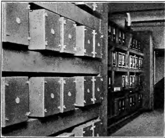
FIG. 4. Part of one of the attic reactor racks, with the reactors in place.
