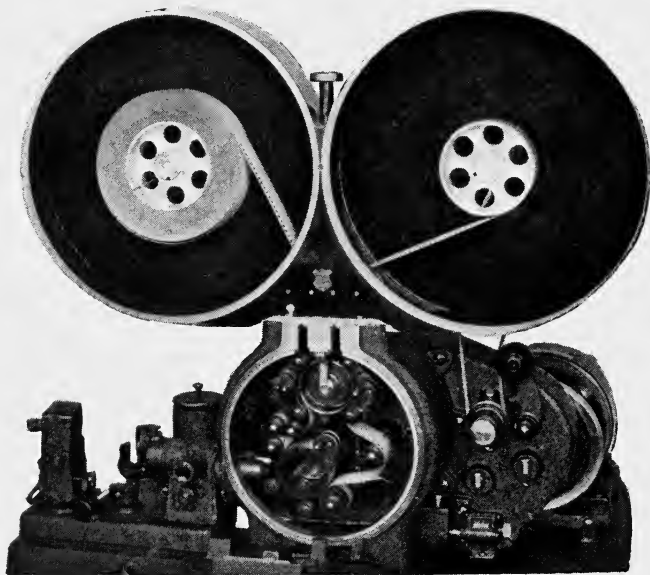
FIG. 12. Recorder, showing normal film loops.
