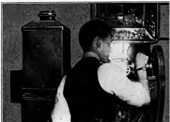
FIG. 1. Television film projector, DuMont station W2XVT.
