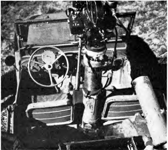
FIG. 9. Mounting of the Mitchell, and the hydraulic pedestal.
