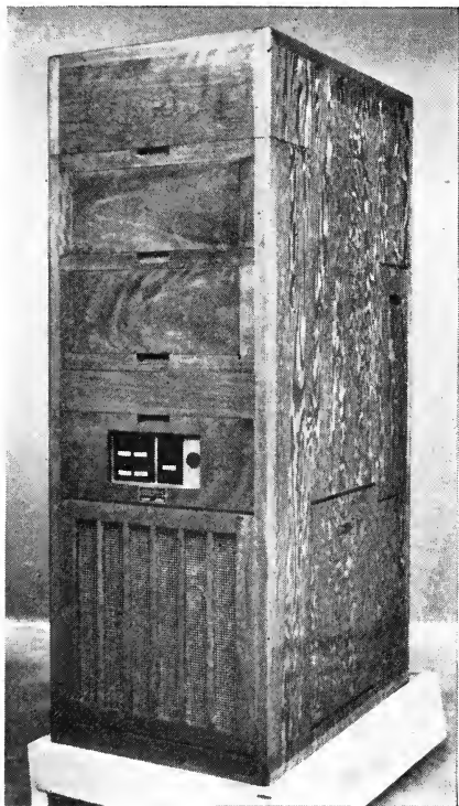
FIG. 5. Drier for two 50-ft reels.
