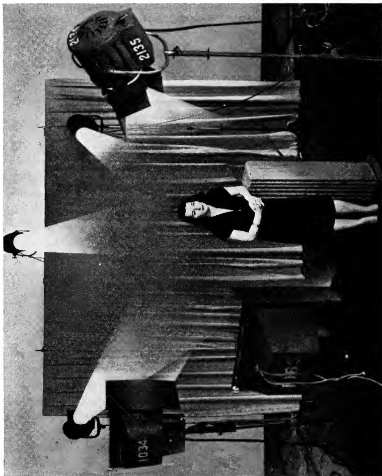
FIG. 1. Standard lighting setup illustrating positioning of the key-light.
