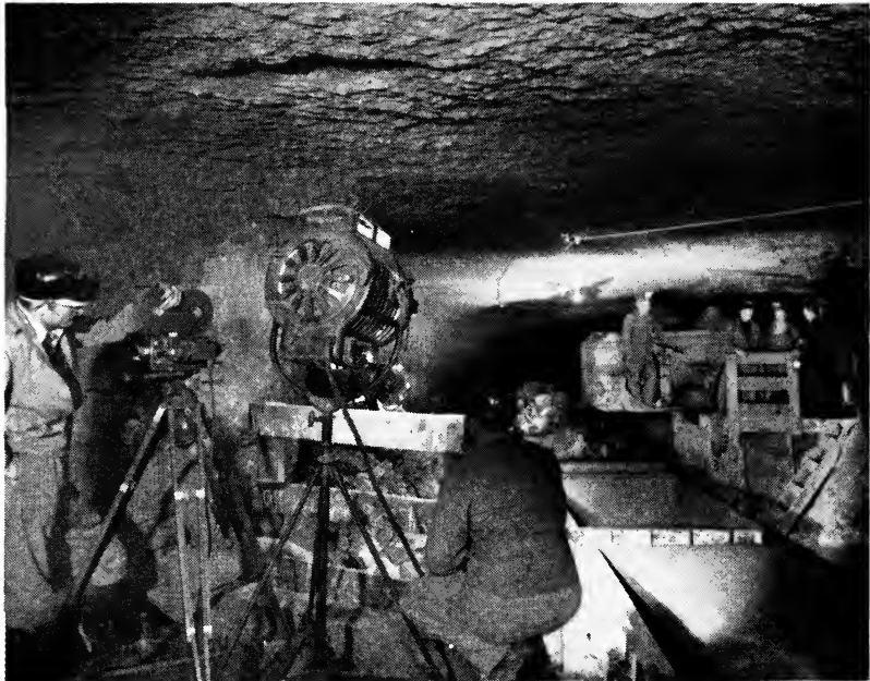
Fig. 2. The main haulage-way in the limestone mine, where the natural ventilation permitted the use of a generator driven by an internal combustion engine; note the Seniors in the center middle distance placed on the rocky ledge to the left of the string of cars ( Photo by Beryl Hawkins ).
