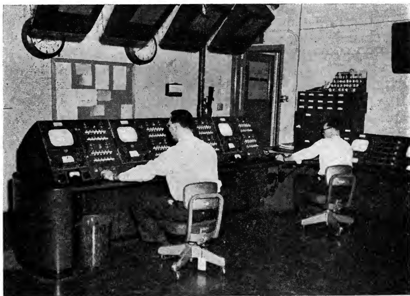
Fig. 4. Master control switching console.
