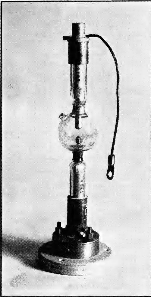
Fig. 1. 1-10-Kw pulse-type compact-source lamp.
