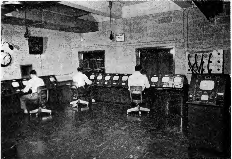
Fig. 3. Camera Control Center with camera cable patch panel at right.
