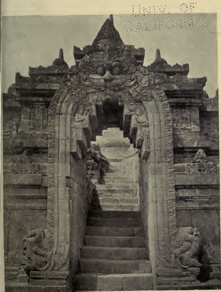
STAIRCASE, BORO BOEDOR
