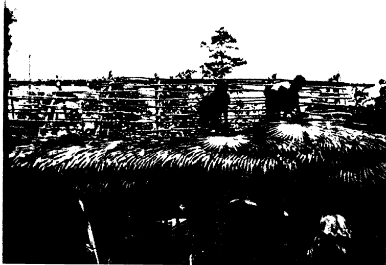
Building our house: Ramon López and his father lashing cross-poles to the roof frame of the shelter they built us beside the Rio Guarabuqui. Afterwards the Jicaques brought palm leaves from the forest and thatched the roof for us, as shown in the other photo.
