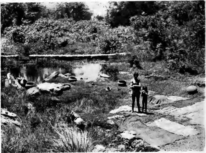
NEAR THE SPILL, ALLAI TANK
