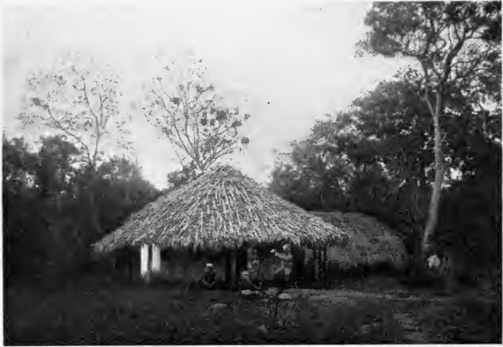
THE BUNGALOW PERIYA KULAM
