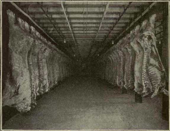
FIG. 82. — Rooms in which meats and other perishable goods are kept are cooled by pipes carrying cold brine.
