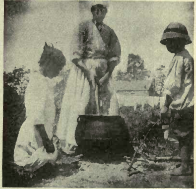
FIG. 107. — The making of soap at home by the cooking of grease and lye.
