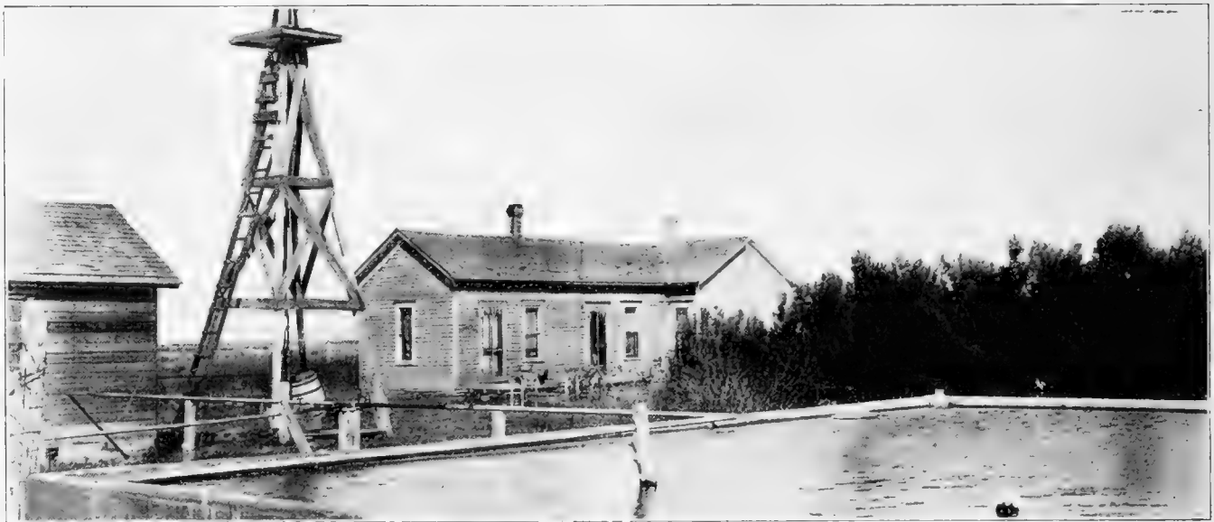
A home-made reservoir, easily and cheaply filled by means of a windmill, will furnish plenty of water to irrigate the garden and supply the household and live stock
