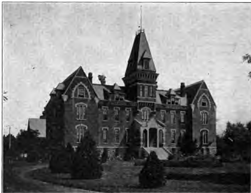
MAIN BUILDING, BOYS' INDUSTRIAL SCHOOL.
