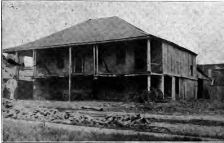
OLD GOVERNMENT BUILDING, FORT SCOTT
