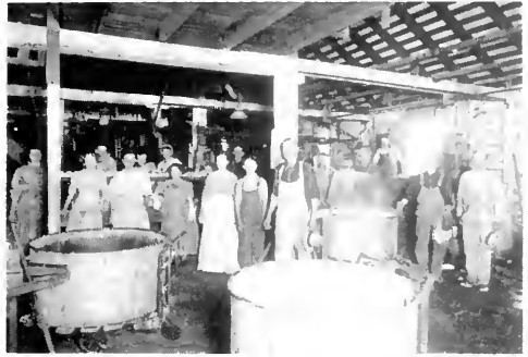
Interior view of Staff Bros. Cannery with employees
