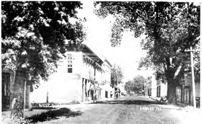
Buena Vista Street, west
