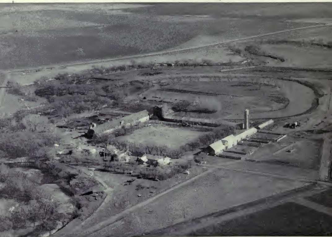
Aerial view of Fort Larned, in Pawnee county.
