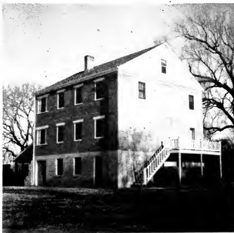
Remaining portion of Iowa, Sac and Fox Presbyterian Mission building near High-
