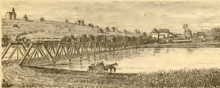
BRIDGE ACROSS THE ARKANSAS RIVER AT LARNED.
