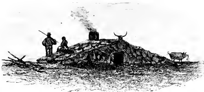
RAWHIDE-FRONTED DUG-OUT—WESTERN KANSAS.
