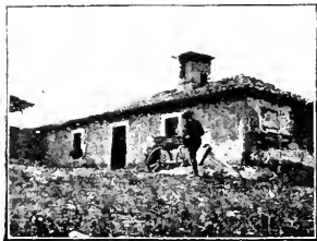
SAN JUAN BLOCK-HOUSE
