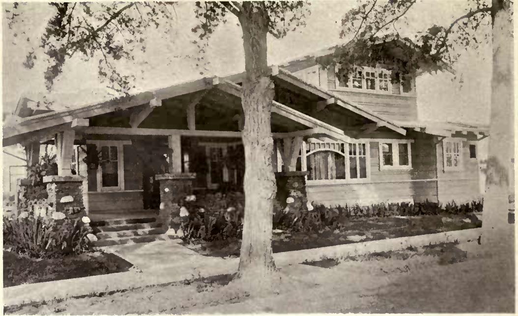
Front view of the Smith bungalow. A happy combination of rough, gray siding and klinker brick with boulders inset.
