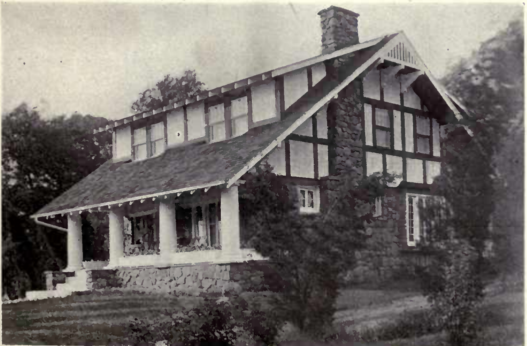
Field stone has been used in the construction of the foundation, first story and chimney walls.
