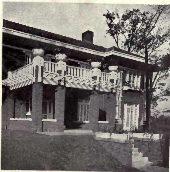
Showing unusual ornamentation of the white terra cotta trim.
