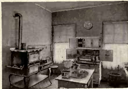
The walls of this kitchen were finished with Carey Ceil-Board, and then papered with sanitary wall-paper.
