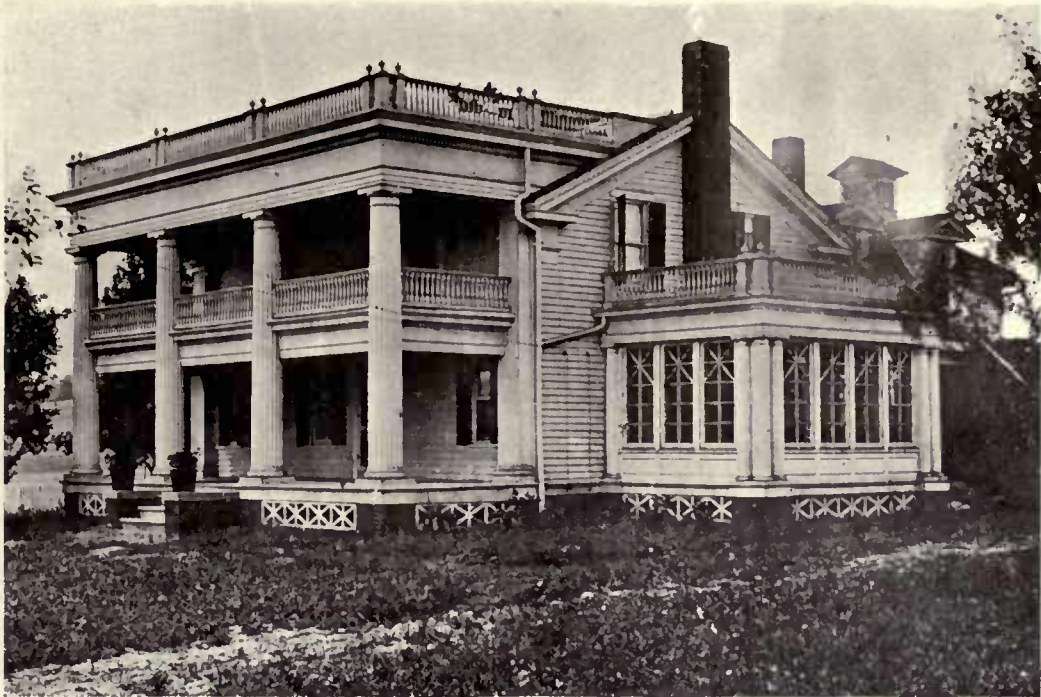
The new house - after being remodeled.
