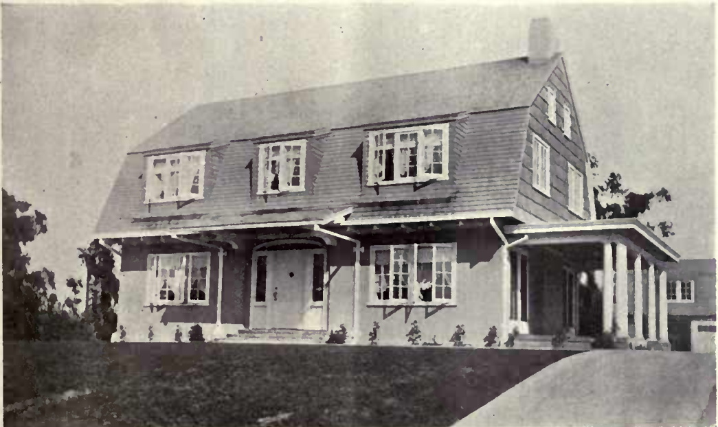
The gambrel roof has an added interest by reason of the dormers.
