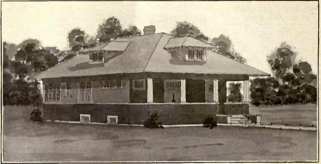
The exterior treatment is cement over metal lath and rough-sawed boards.
