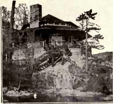
Stained with Cabot's Shingle Stains Davis, McGrath & Shepard, Architects, N. Y.
