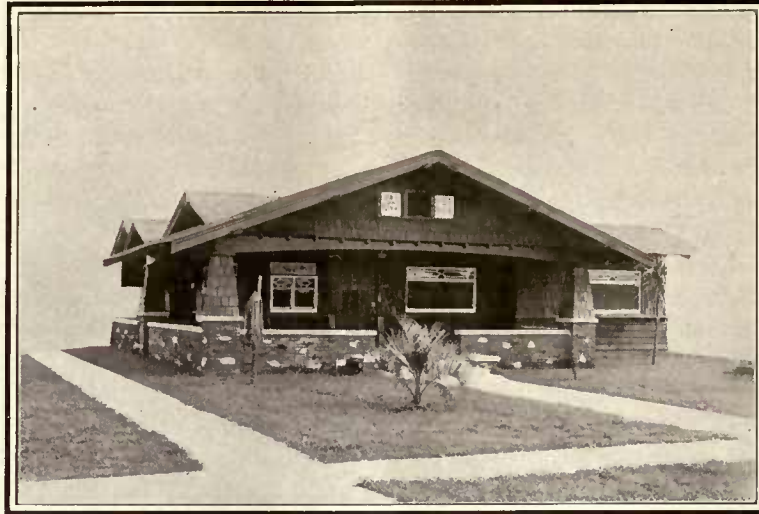
An open effect to the porch is gained by a single span between corner pillars.
