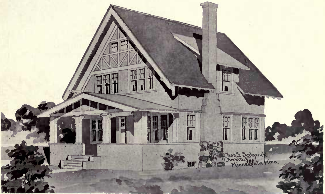
The walls are cemented on the outside. The gables showing half timbers and verge boards.—C. S. Sedgwick, Architect.
