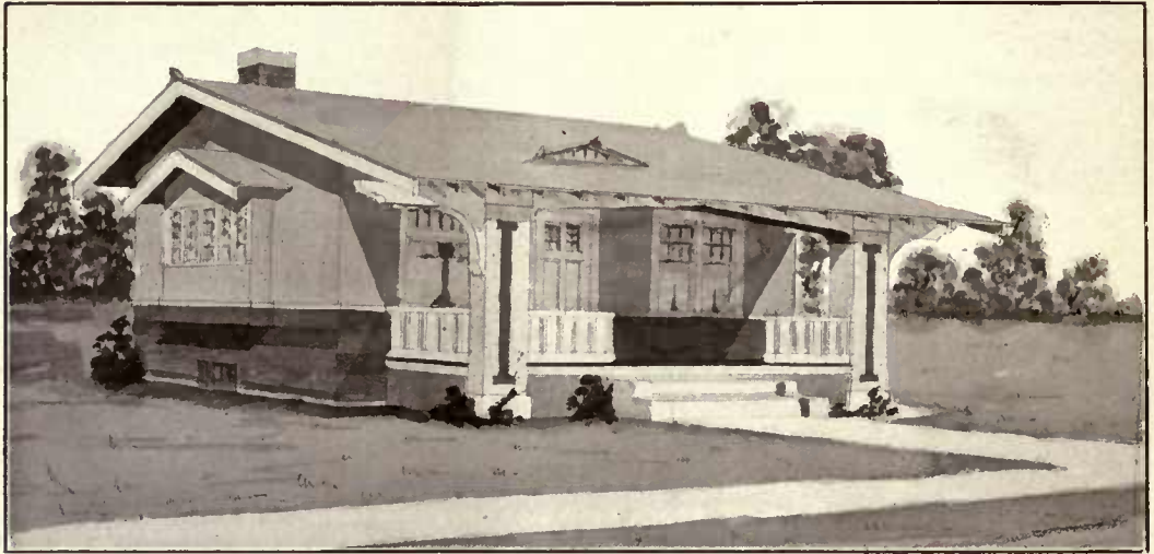
Wide, rough-sawn drop siding, and rough-cast cement above are used for the exterior walls.
