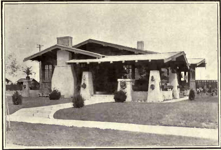
The cement makes an excellent background. Jud Yoho, Archt.
