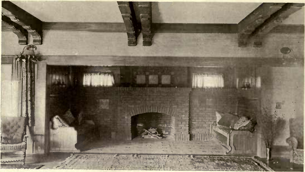
The brick hearth is the width of the seats.
