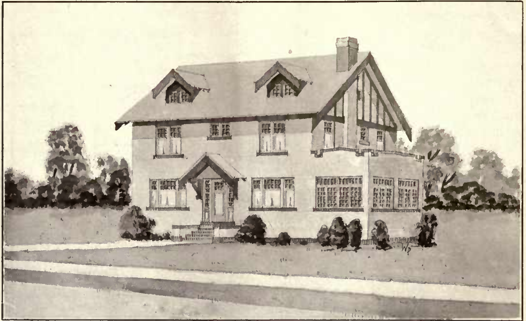
Walls are of hollow tile faced with brick, with rough-cast cement plaster and half-timbers in gables.
