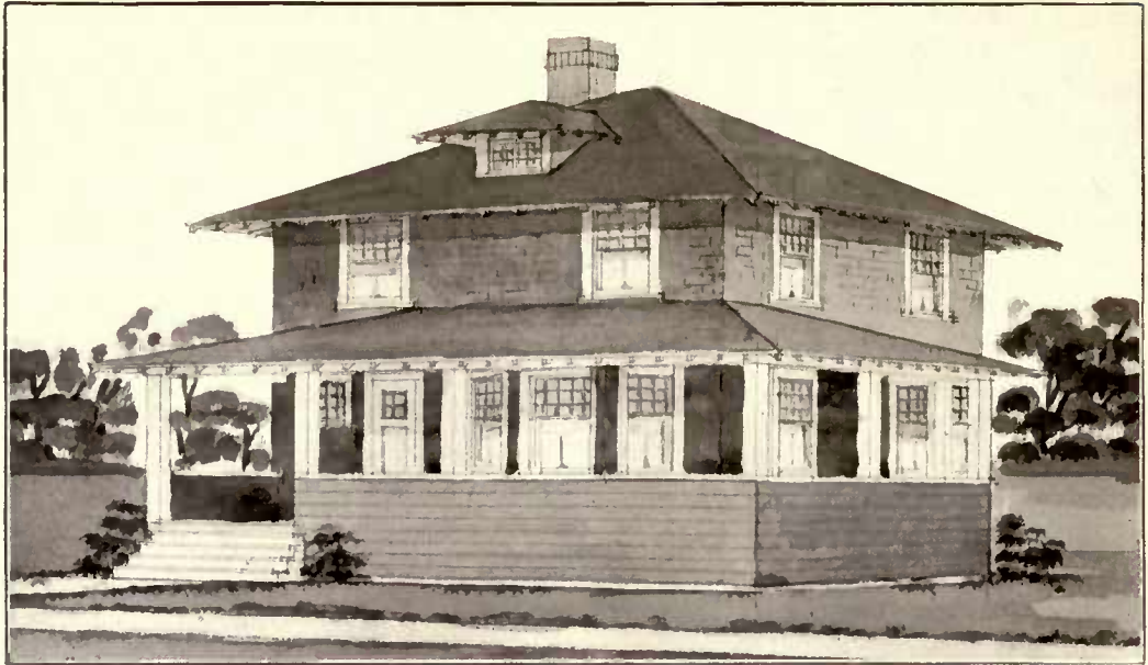
Treatment of exterior walls in rough-sawn drop siding, used up to first story sills and shingles above.
