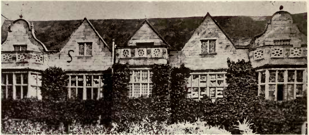
The window openings are many and large.
