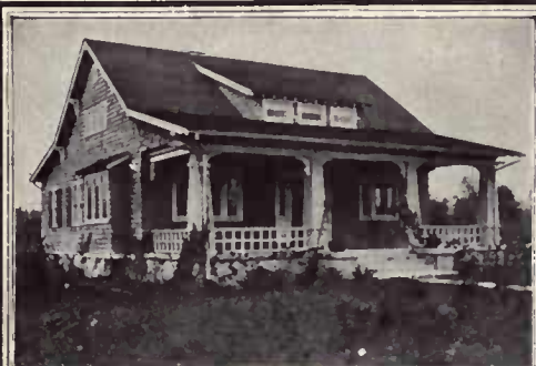
Stained with Cabot's Shingle Stains. Hollingsworth & Bragdon, Arch'ts, Cronford, N. J.
