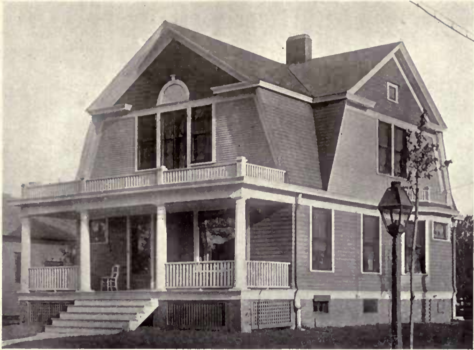
This cottage would nicely accommodate a family of five or six. F. E. Colby, Architect.
