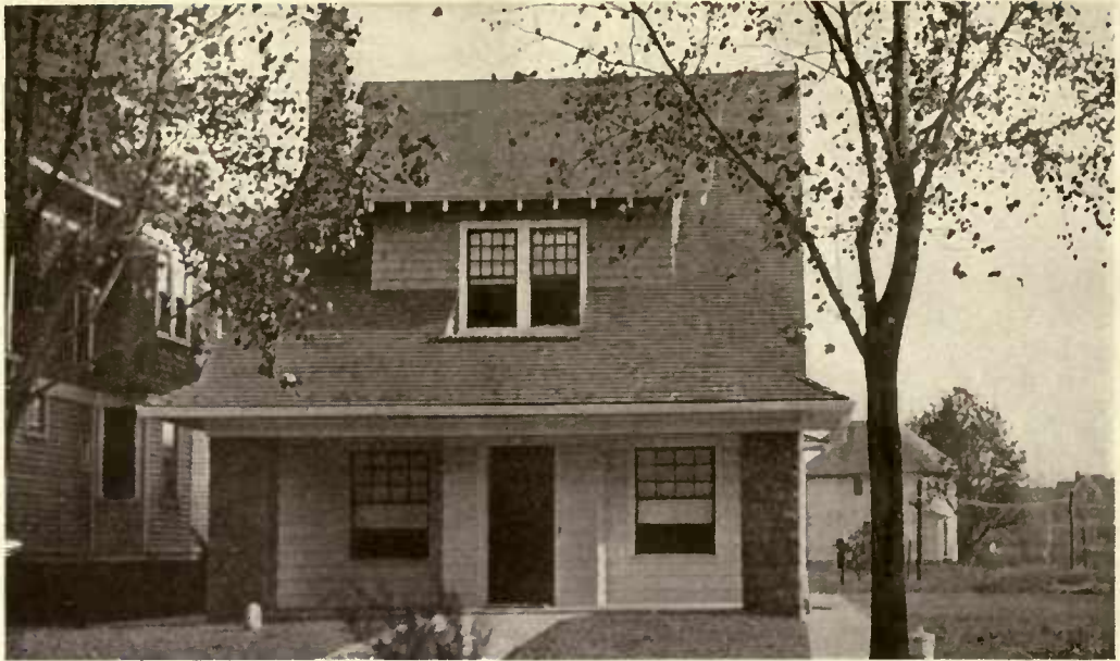
The stone porch piers give an interest.
