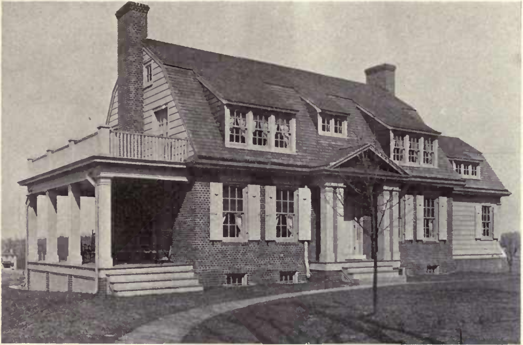
A present-day Colonial cottage in Pennsylvania. The gambrel roof and Dutch dormers make plenty of space upstairs.
