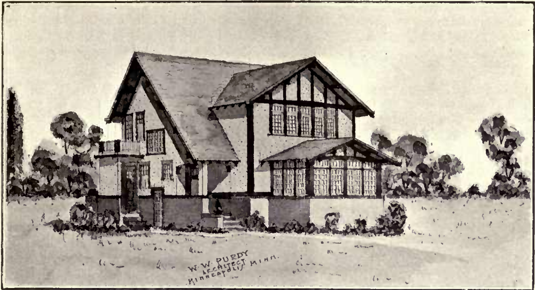
The exterior walls are brick with cement plaster and half timbers above.—W. W. Purdy, architect.
