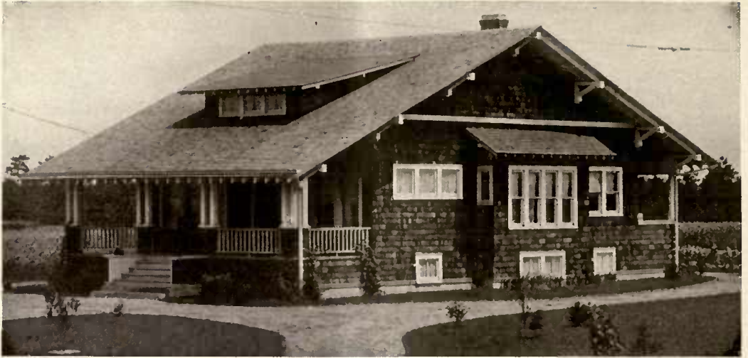
The house has a surprising amount of room.
