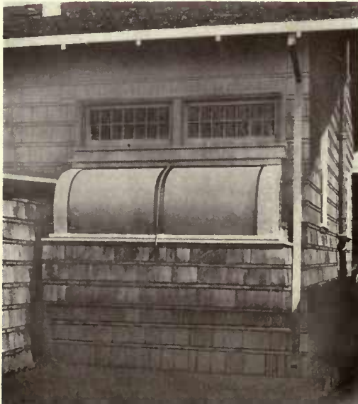
Exterior view, showing appearance in building.
