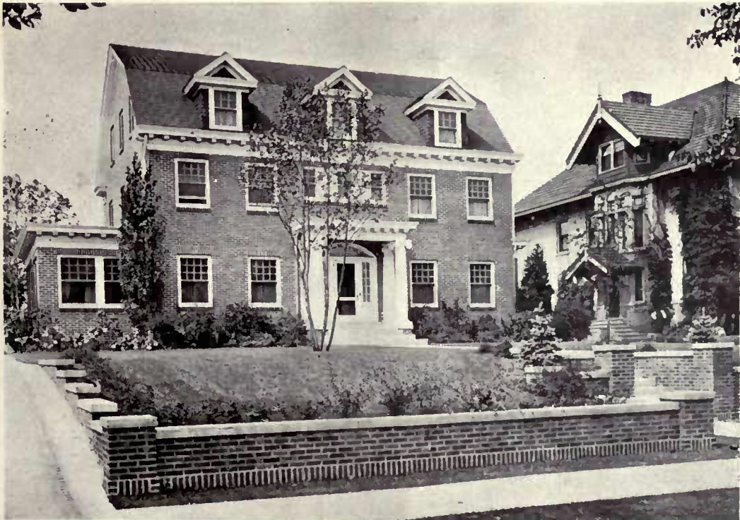
Residence of Mr. William S. Jones, Minneapolis, Minn. Designed by Louis S. Childs, Architect.
