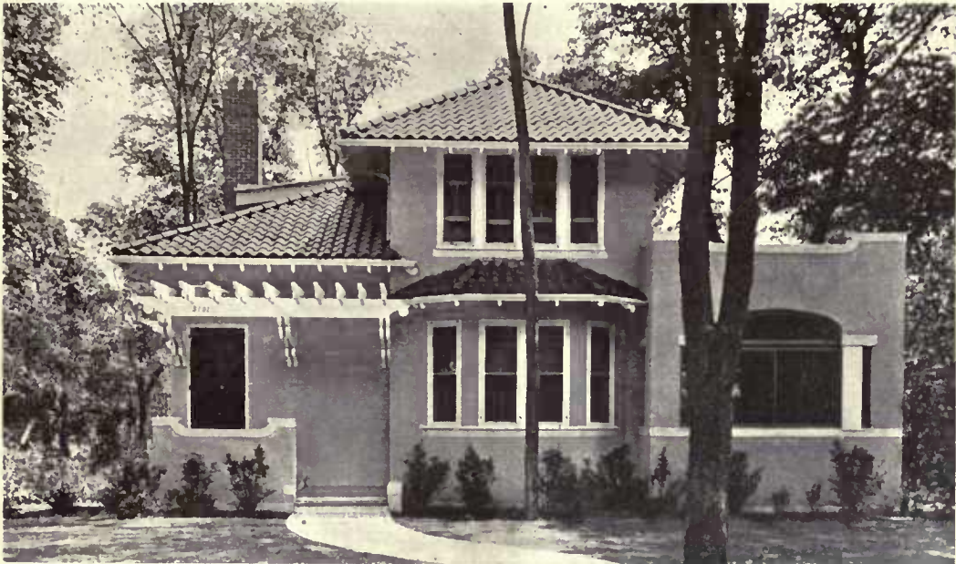
The roof gives the key to the design.
