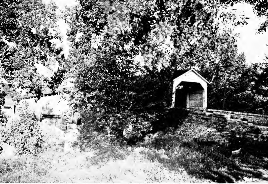
COVERED BRIDGE, CYNTHIANA
