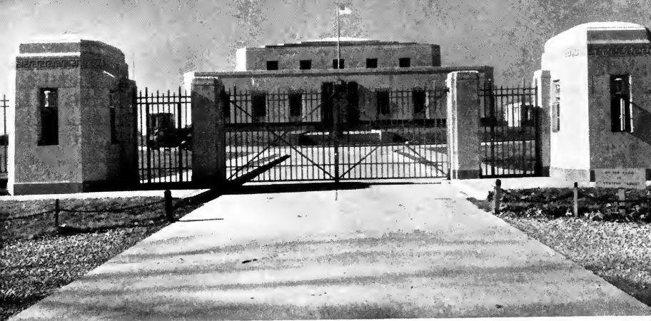
GOLD DEPOSITORY, CAMP KNOX
