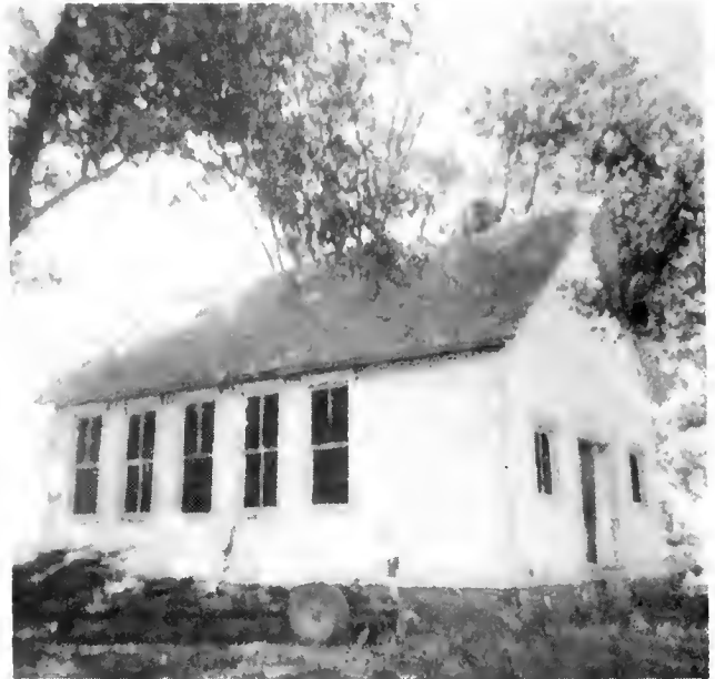
LONG BRANCH SCHOOL — Picture taken just before tearing it down.
