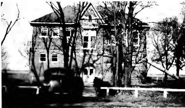
KTHS — Two-story building
