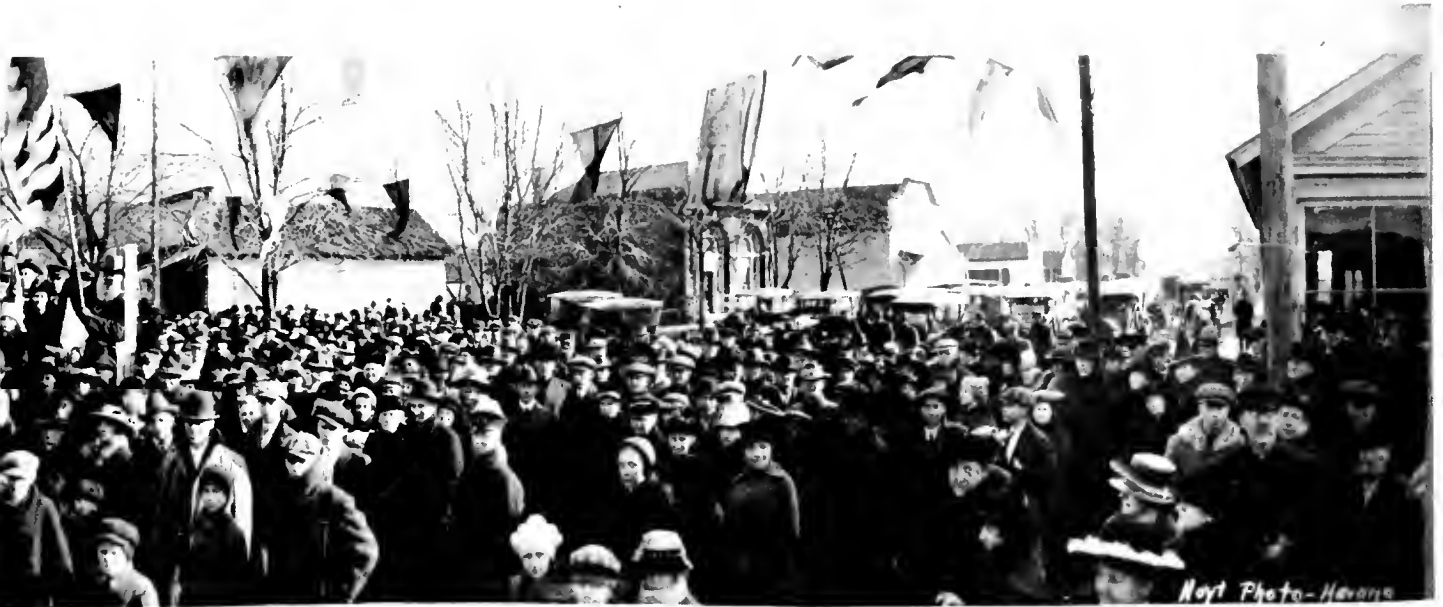
This panoramic view of downtown Kilbourne answered several questions about the location of business places during this period and — raised a few more that are unanswered.
