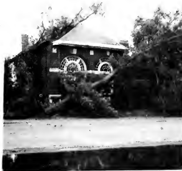
BANK OF KILBOURNE — No record of dates. TORNADO DAMAGE — JUNE, 1964
