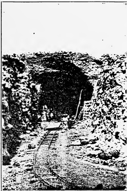
Number 62.—TUNNEL. One of 15 on the Colima Line.
