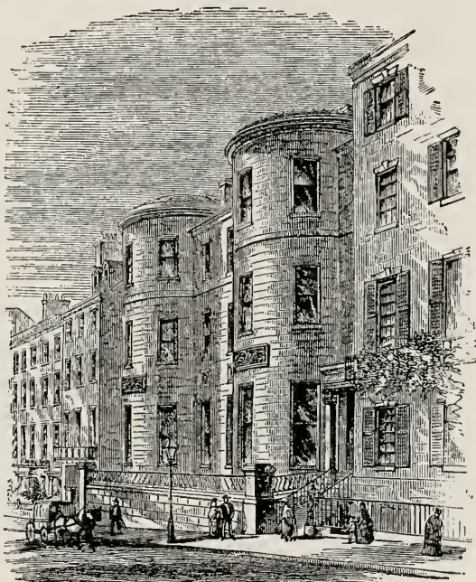
Somerset Club House, Beacon Street.
