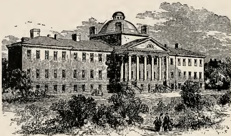
The Massachusetts General Hospital, Blossom Street.
