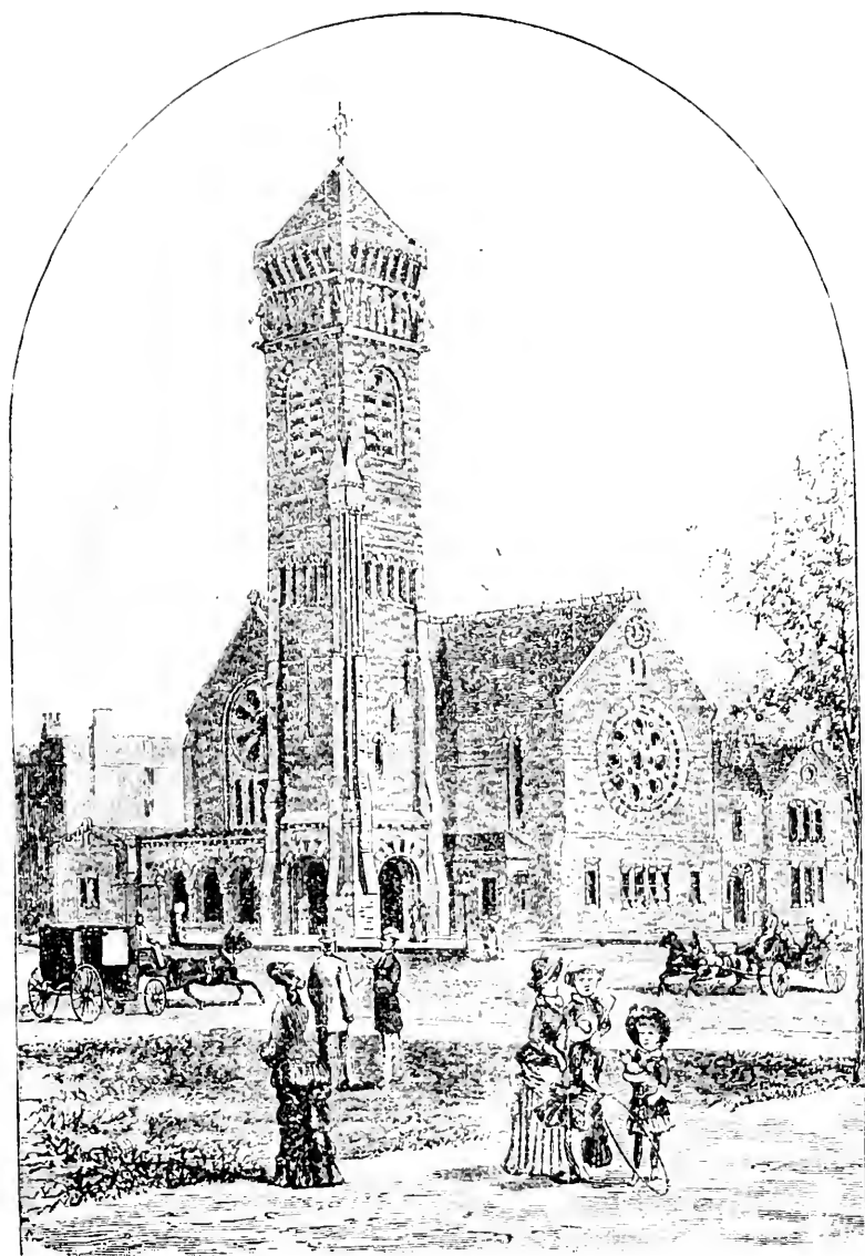
FIRST BAPTIST CHURCH, COMMONWEALTH AVENUE.
