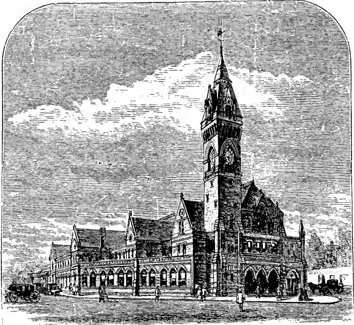
Boston and Providence Railroad Depot, Columbus Avenue.
