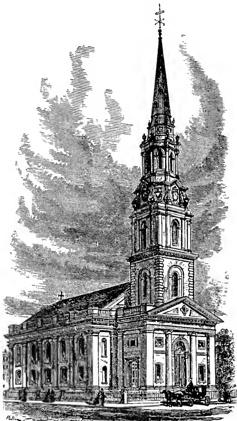
The Arlington-street Church, corner of Boylston Street.
