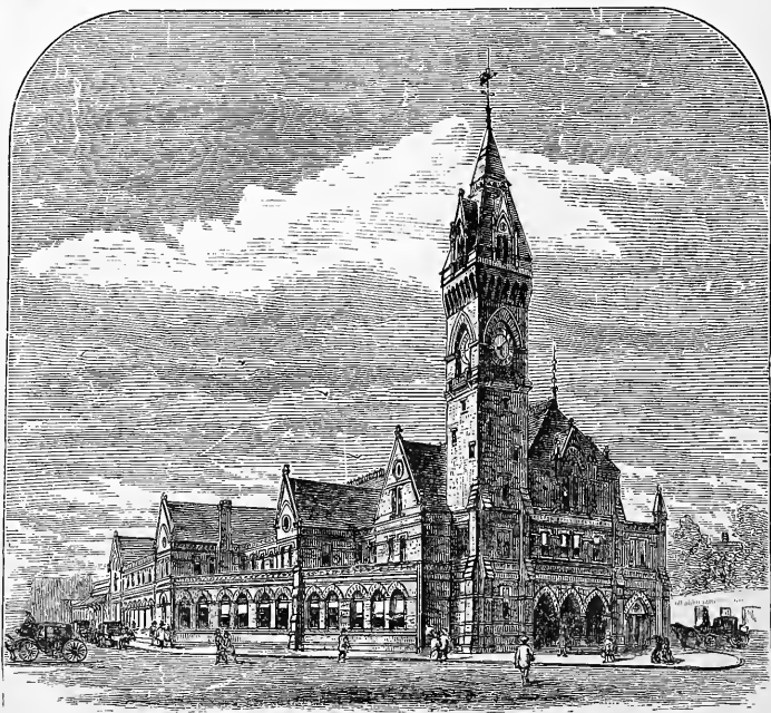
Boston and Providence Railroad Depot, Columbus Avenue.
