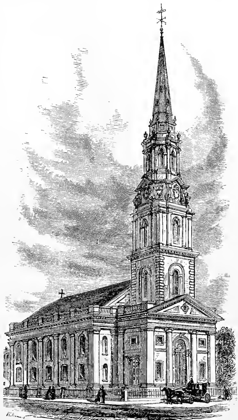
The Arlington-street Church, corner of Boylston Street.
