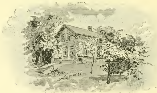
Residence of J. R. Prescott, Linwood Park, Newtonville, Mass. Heated by one Anthony Steel Plate Furnace.
