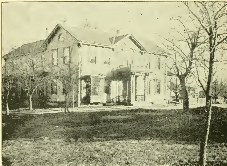
Edwin W. Gay's Residence, Waverley Avenue and Church Street.
