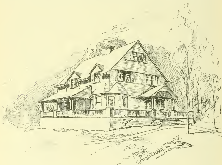
The New Dresser House at Waban.
