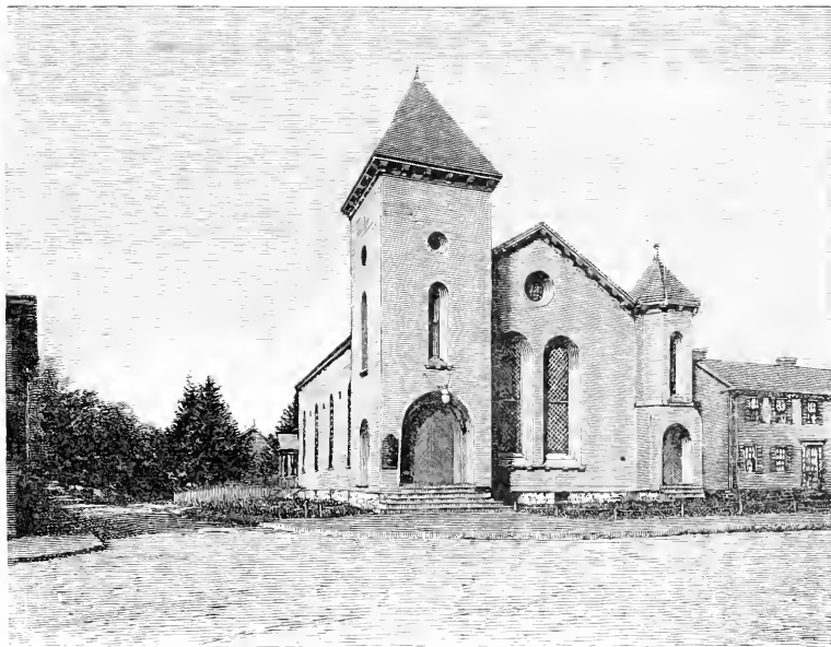
Associates' Hall, Centre and Pelham Streets, Newton Centre.
