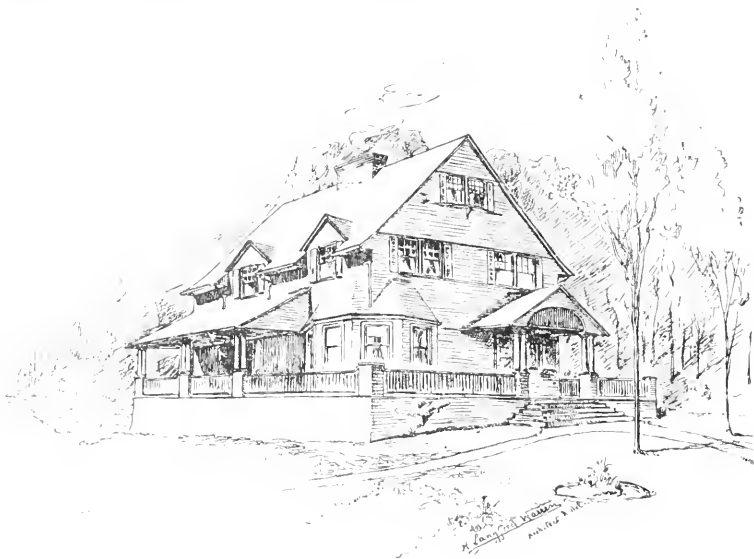
The New Dresser House at Waban.
