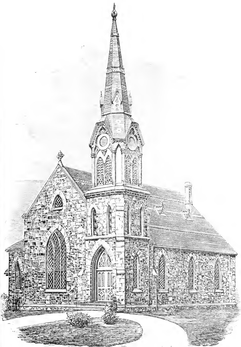
THE UNIVERSALIST CHURCH. Washington Park, near Walnut Street, Newtonville,
