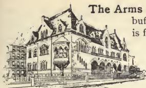
EVANSVILLE : U. S. COURT-HOUSE AND POST-OFFICE.
