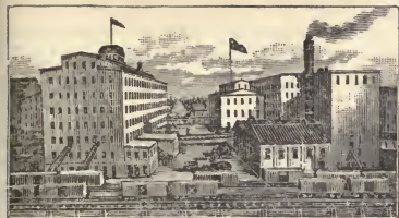
MINNEAPOLIS: THE WASHBURN-CROSBY COMPANY THE "WASHBURN" FLOURING MILLS.
