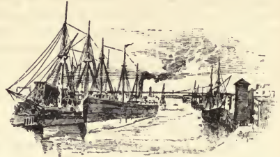
CLEVELAND : IRON-ORE VESSEL OF PICKANDS, MATHER & CO.
