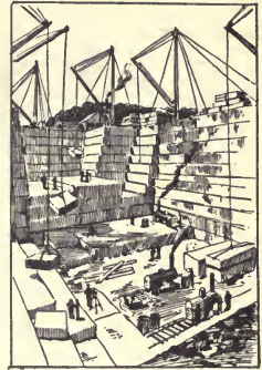
NORTH AMHERST; QUARRY NO. 6. CLEVELAND STONE CO.
