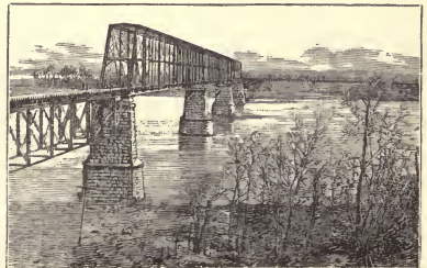
SIBLEY BRIDGE: MISSOURI RIVER.
