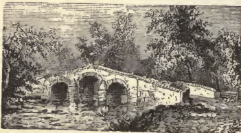
ANTIETAM: BURNSIDE'S BRIDGE.
