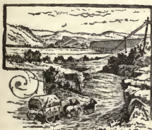
TEXAS & PACIFIC RAILWAY : PALO-PINTO BRIDGE.
