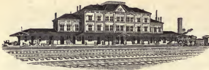
HOUSTON; HOUSTON &amp; TEXAS CENTRAL RAILROAD DEPOT.
