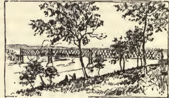
FORT LEAVENWORTH : MISSOURI-RIVER BRIDGE.
