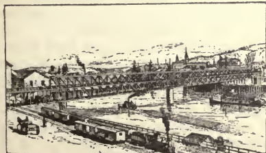
PORTLAND : STEEL BRIDGE OVER THE WILLAMETTE.
