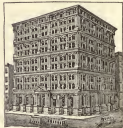
ST. LOUIS: EQUITABLE BUILDING. GENERAL OF- FICES MISSOURI PACIFIC RAILROAD.
