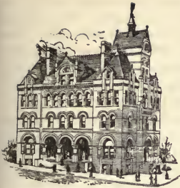
MARQUETTE : THE POST-OFFICE.
