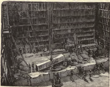
TATE: GEORGIA MARBLE COMPANY'S DEEP QUARRY.
