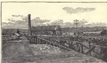
TOWER : MINNESOTA IRON CO.
