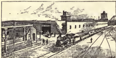
MEMPHIS : WAREHOUSE NO. 1, OF HILL, FONTAINE &amp; CO.
