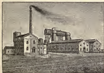
BESSEMER : DE BARDELEBEN COAL AND IRON CO.
