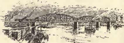
ST. LOUIS: THE MERCHANTS' BRIDGE.
