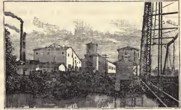
LOUISVILLE : WESTERN CEMENT WORKS.
