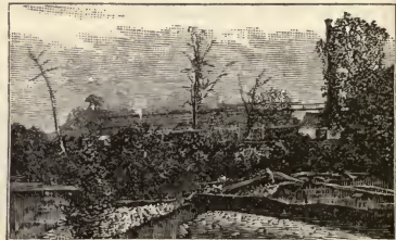
LOUISVILLE: WESTERN CEMENT WORKS.
