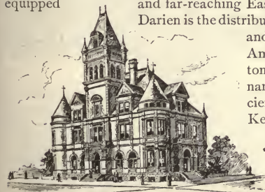
MACON : U.-S. COURT-HOUSE AND POST-OFFICE.
