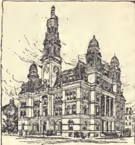
MINNEAPOLIS : THE POST-OFFICE.
