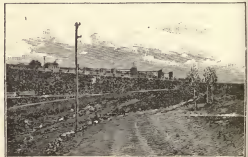
TOWER: MINNESOTA IRON CO.
