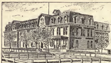
EXCHANGE BUILDING: KANSAS CITY STOCK YARDS.
