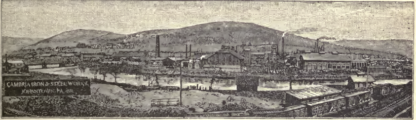
JOHNSTOWN : THE CAMBRIA IRON WORKS.
