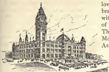
MINNEAPOLIS: EXPOSITION BUILDING.
