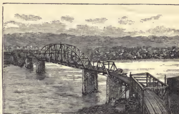
WHEELING : BRIDGE ACROSS THE OHIO.
