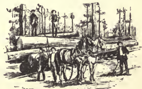
CUTTING TIMBER ON THE LINE OF THE HOUSTON & TEXAS CENTRAL RAILROAD.
