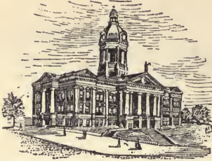
SEATTLE: KING-COUNTY COURT-HOUSE.
