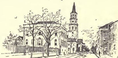
CHARLESTON : ST.-MICHAEL'S CHURCH.
