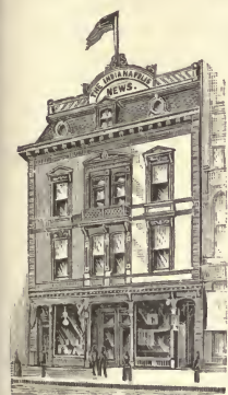
INDIANAPOLIS : INDIANAPOLIS NEWS BUILDING.
