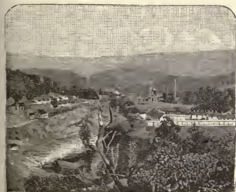
RIISING FAWN FURNACE : GEORGIA MINING, MANUFACTURING AND INVESTMENT COMPANY.
