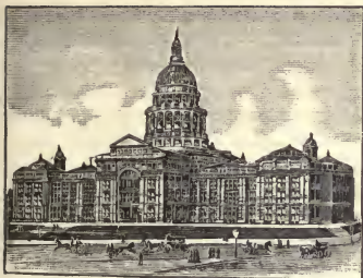
AUSTIN : STATE CAPITOL. BUILT BY THE CAPITOL FREEHOLD AND INVESTMENT COMPANY.
