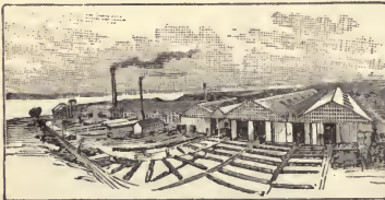
EDGE MOOR BRIDGE WORKS.
