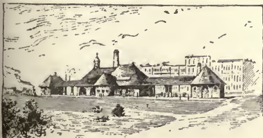
KALAMAZOO : MICHIGAN-CENTRAL RAILROAD STATION.
