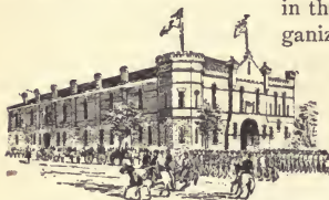
PORTLAND : FIRST REGIMENT ARMORY.
