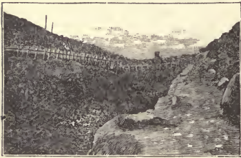
TOWER: MINNESOTA IRON CO.
