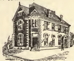
BESSEMER : OFFICE OF THE BESSEMER LAND AND IMPROVEMENT CO.
