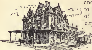
WILMINGTON : P. W. &amp; B. STATION.
