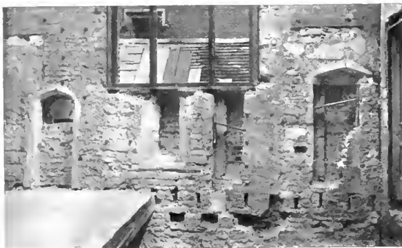
Fig. 8. Doors and windows. North end.
