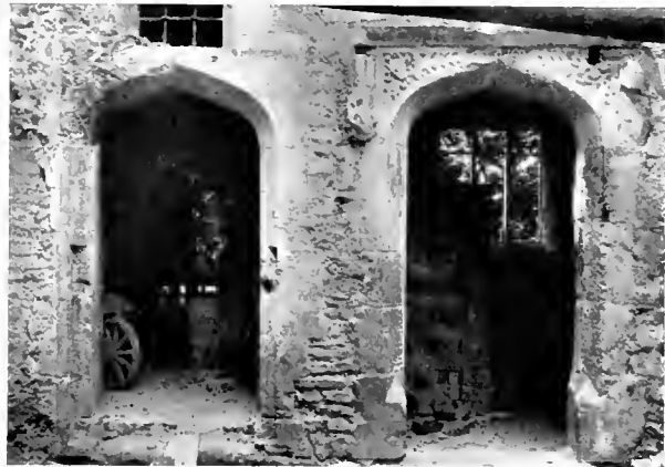
Fig. 14. Doors towards the Cloister.
