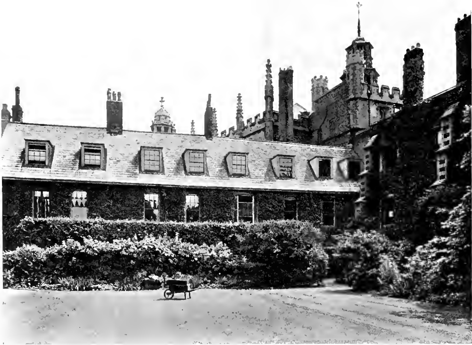
Fig. 2. Bowling Green Front, before the recent works.
