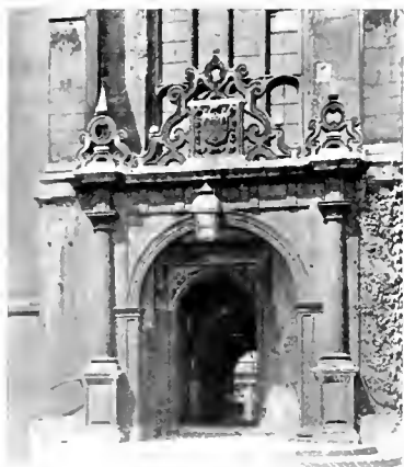
Fig. 23. Doorway in Neville's Hall.
