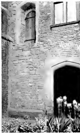
Fig. 21. Entrance door to 1st floor chamber adjoining St John's boundary.
