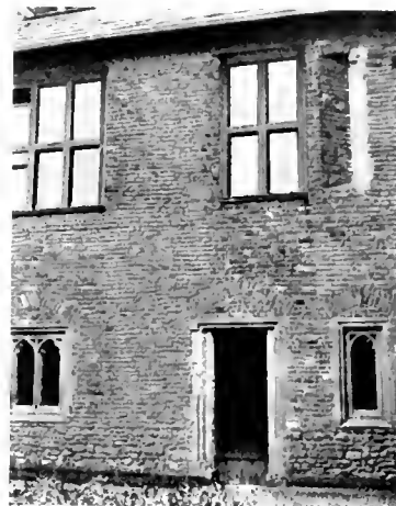
Fig. 15. Blocked doorway to the Bowling Green.
