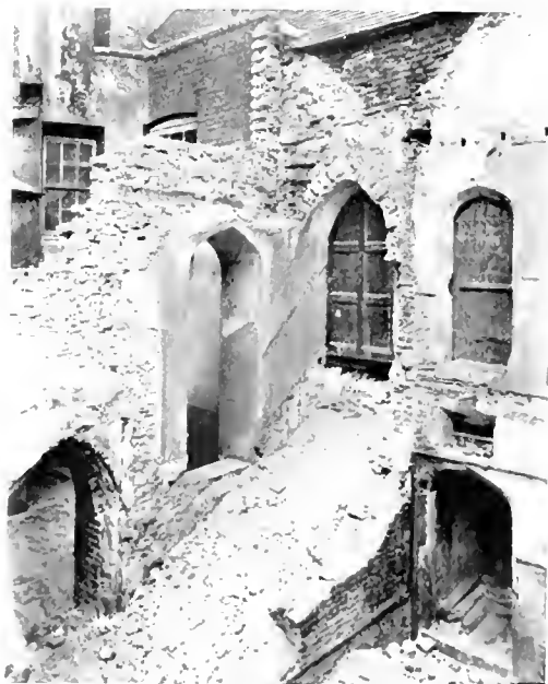
Fig. 16. Remains of the Master's Stairs.
