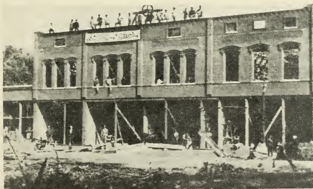
Rebuilding the opera house after the fire of 1903.
