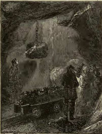
BOTTOM OF A SHAFT
