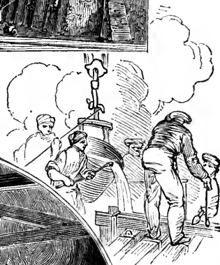
CASTING PIPES
