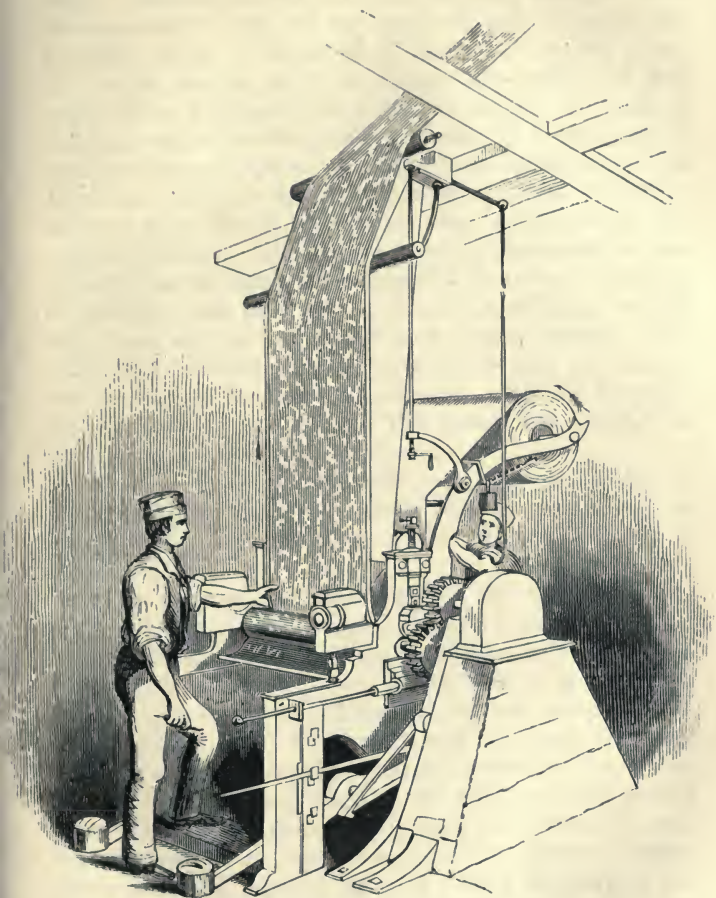
Calico-printing by Cylinder.
