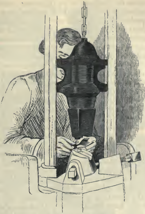
Stamping the eye of a needle.
